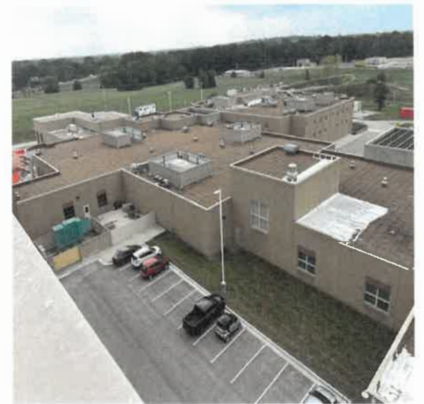
Overall view of existing roof system.
