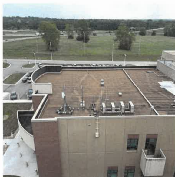
Overall view of existing roof system.
