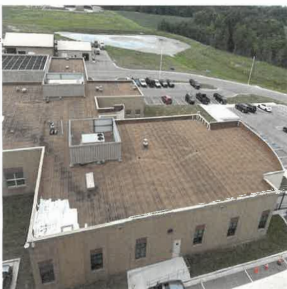
Overall view of existing roof system.
