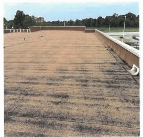
Field of roof has moderate granule loss but in fair condition.
