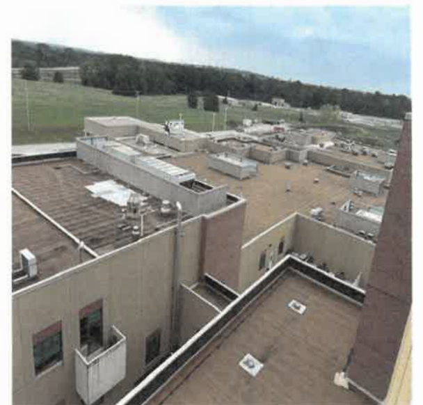
Overall view of existing roof system.
